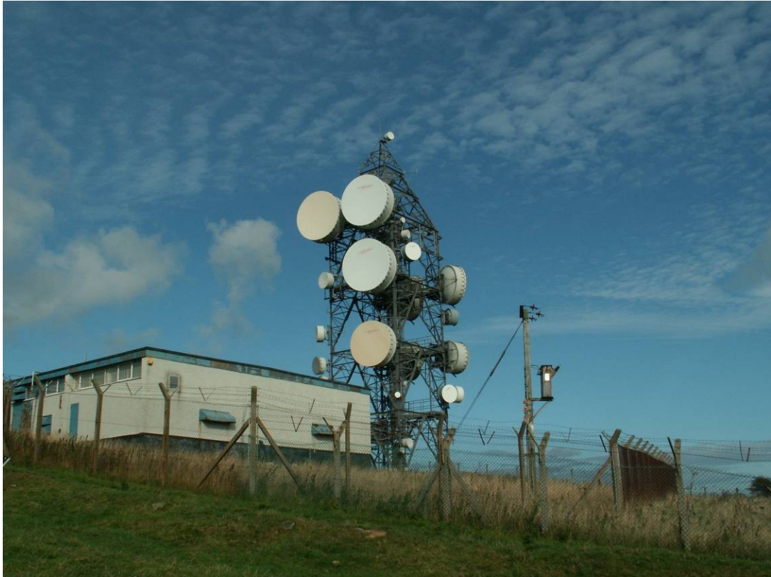
Photograph 6 – Dalton Radio Mast
