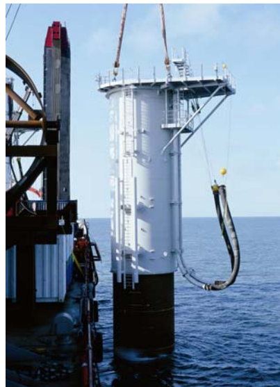
Figure 3 : Monopile Foundation, Arklow Bank
