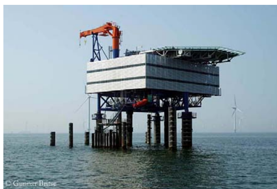
Figure 5 : Transformer Station, Horns Rev
