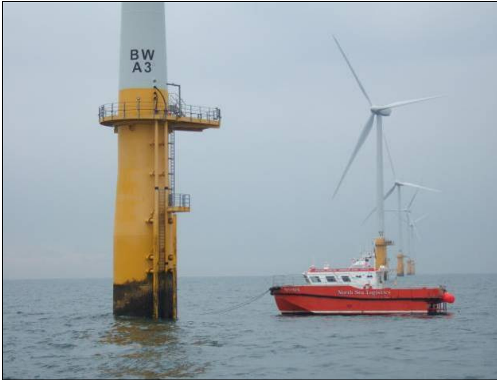
Service vessel at the Kentish Flats
